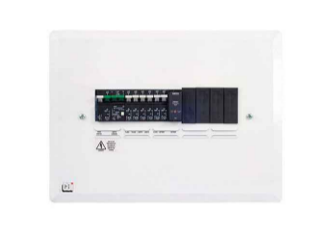
TYPICAL DISTRIBUTION BOARD
